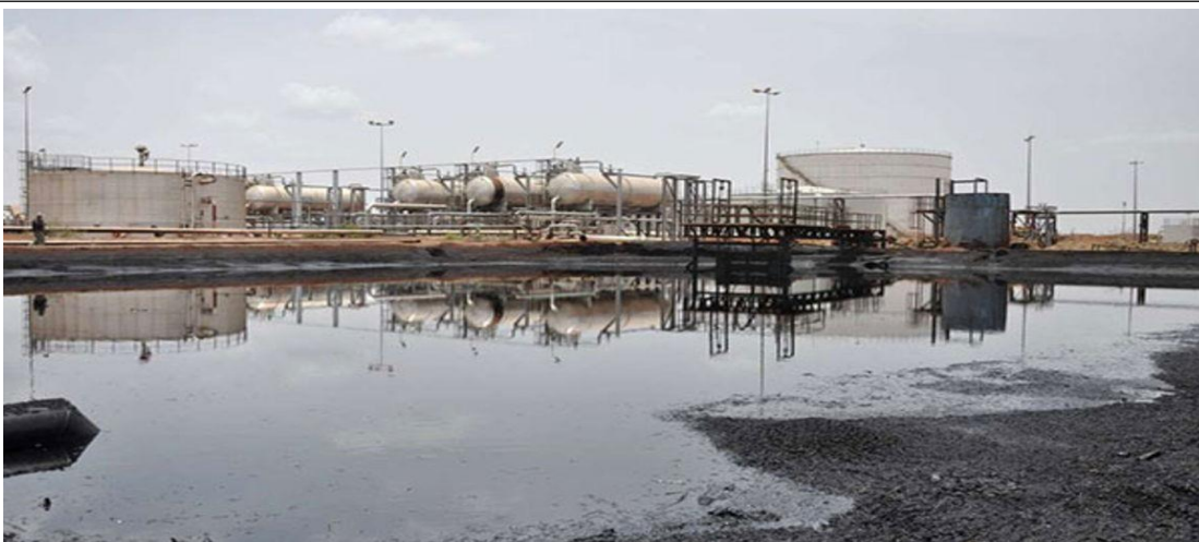
This is the meeting point of all the networks of pipelines in Unity Oilfields coming from Tharjiath oilfields and other areas of Unity oilfields. From here, the main pipeline takes the oil to Heglig oilfields from which it proceeds to Port Sudan (Red Sea)
