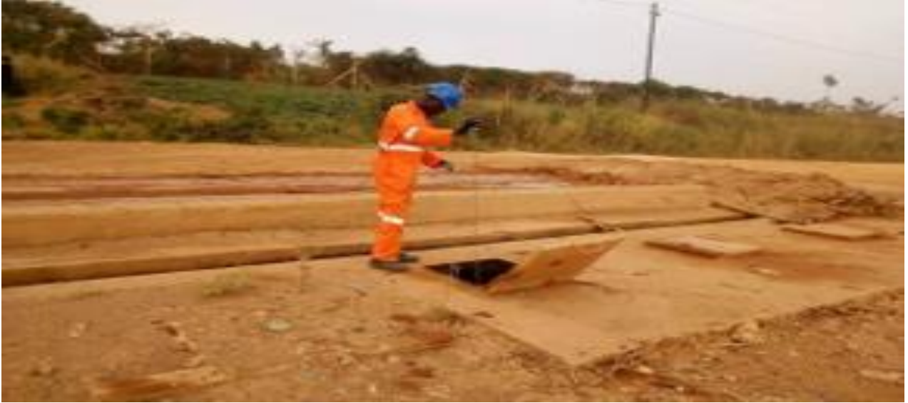
Figure 4.12: Septic Monitoring at Kabaale Airport Source: Primary Data
