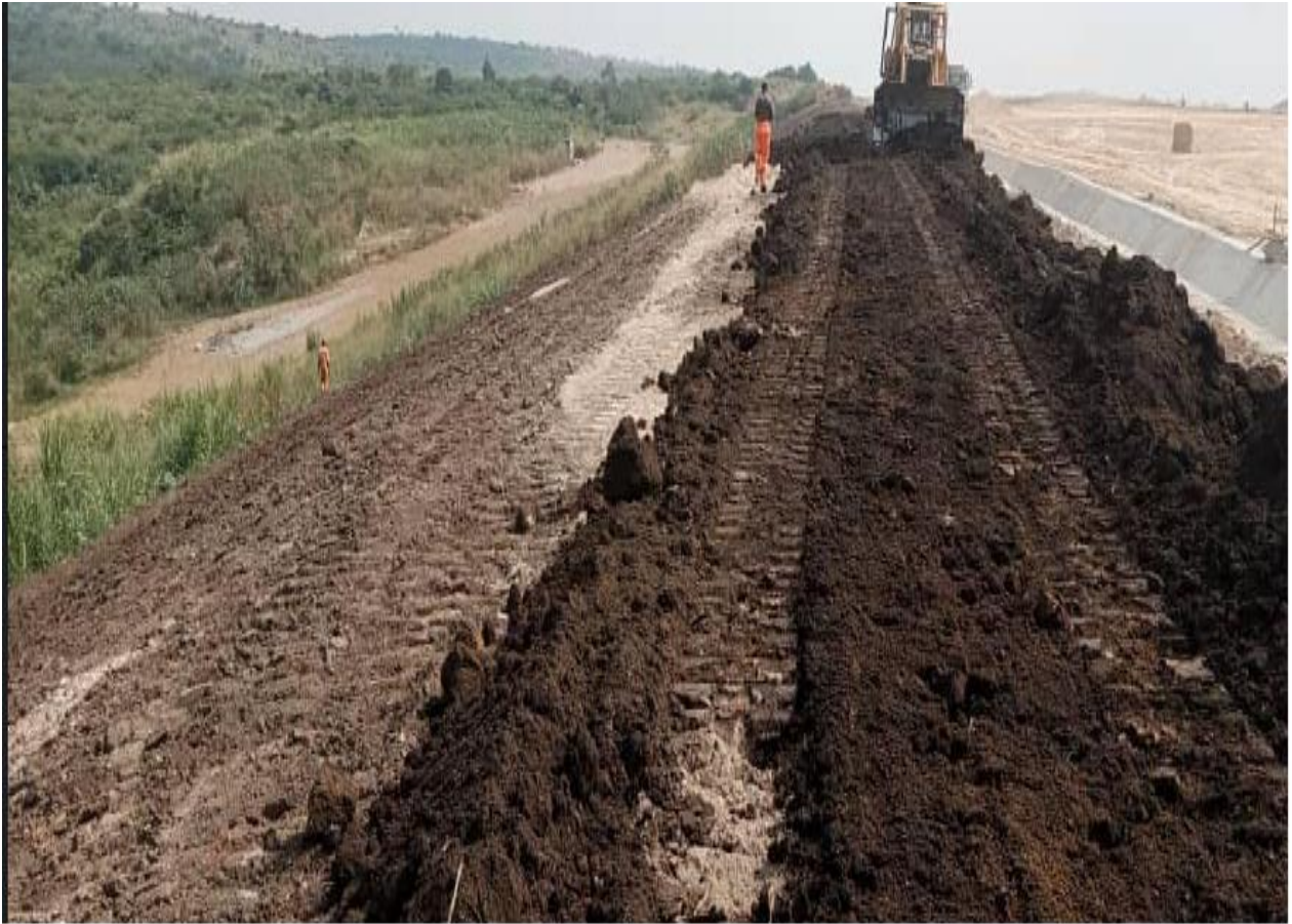
Figure 4.13: Topsoil reinstatement at Kabaale Airport Source: Primary Data
